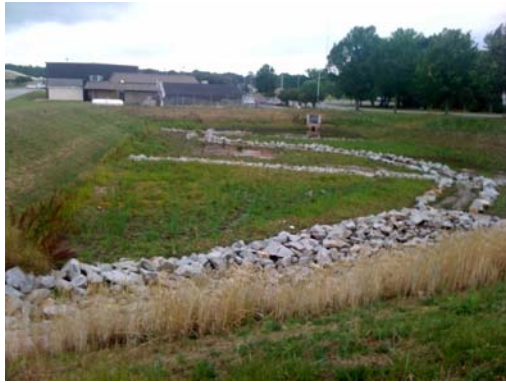
Storm Water Wetland
